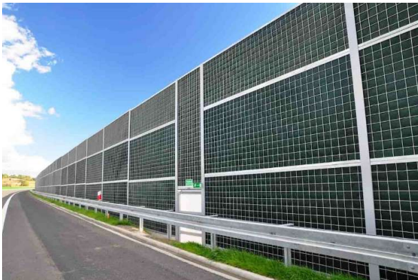
Figure 2. Noise barriers manufactured by Weldon Sp. z o.o.
